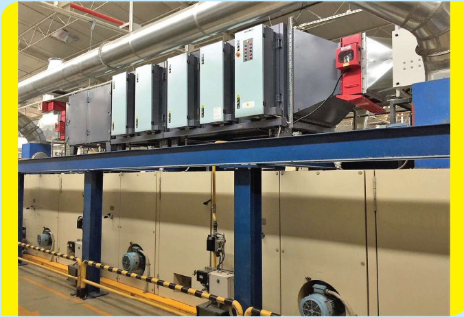
HOT WATER RECOVERY SYSTEM
