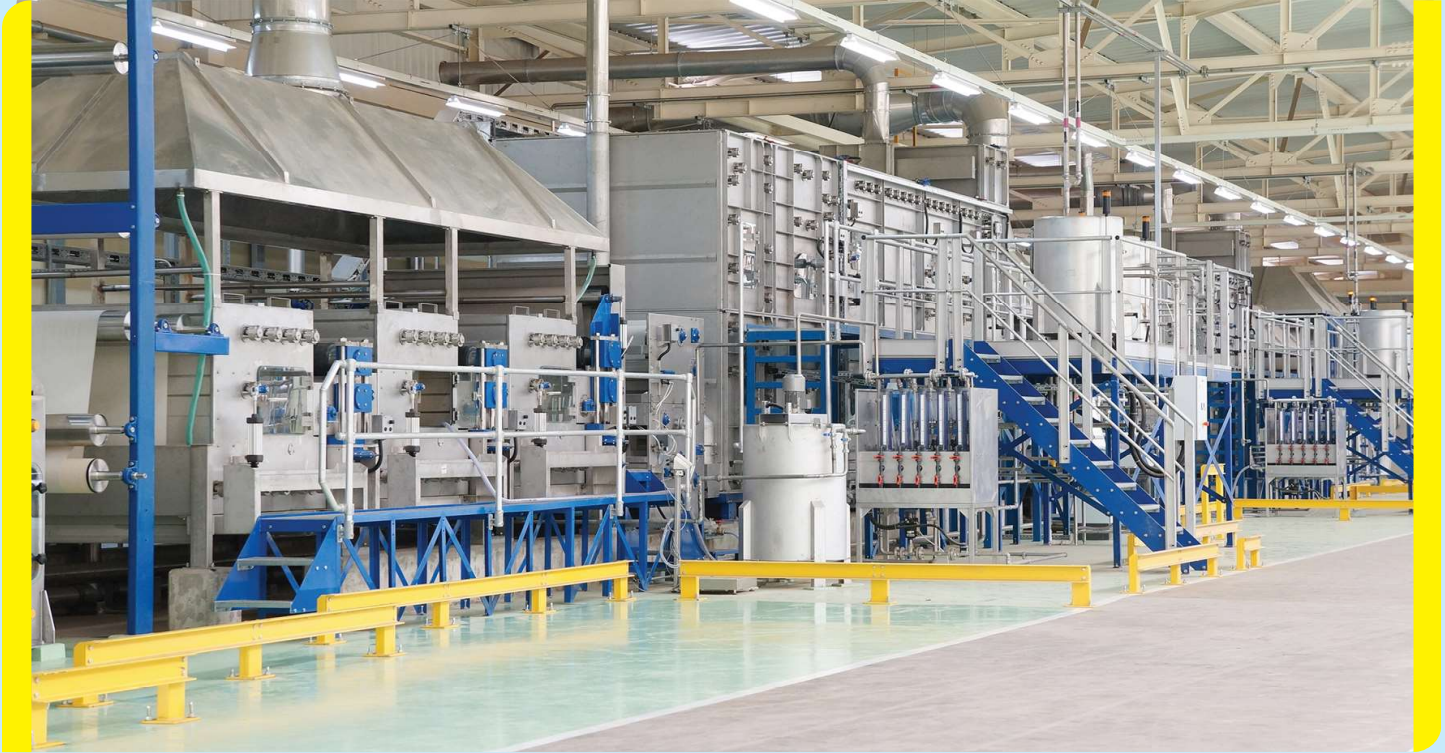
CONTINUOUS SCOURING BLEACHING RANGE
