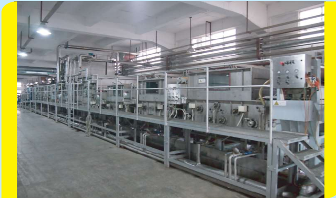
OPEN WIDTH SCOURING BLEACHING
